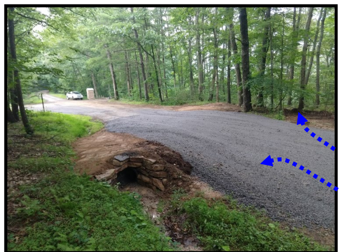
WITH GRADE BREAK (and associated crosspipe) – Interruption in slope redirects flow and guides water to a pipe inlet and a turnout.
